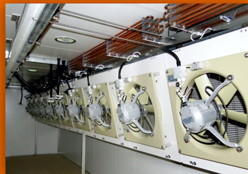
Fan-boards easily lowered for maintenance
