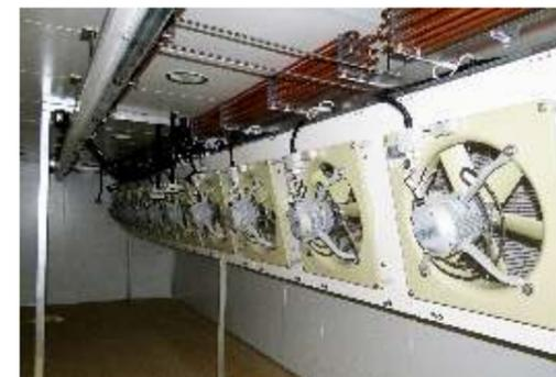
Fan-boards easily lowered for maintenance
